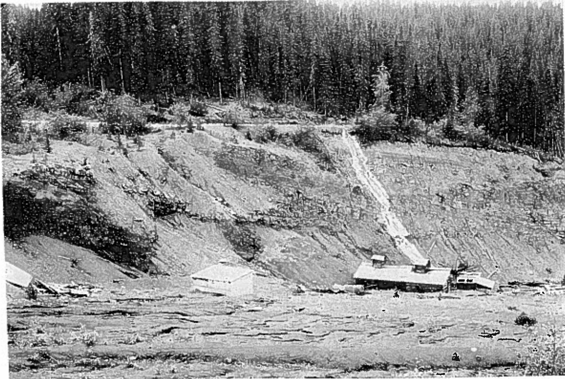
Figure 17. Coal and overburden section near old mine entrance at No.12 level (STOP 8).
