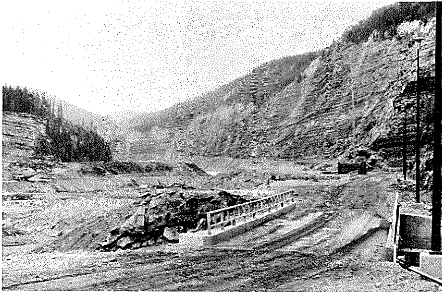
Plate 3: Gething Formation viewed from toe of Bennett Dam looking downstream toward Gething Creek.
